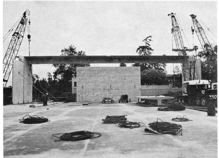
CONSTRUCTION PROGRESSES—Large cranes lift first mammoth roof beam—116 feet long and 54 tons—into place. Left, 38,000-pound wall panel of prestressed concrete is bolted in position.
