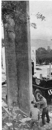
CONSTRUCTION PROGRESSES—Large cranes lift first mammoth roof beam—116 feet long and 54 tons—into place. Left, 38,000-pound wall panel of prestressed concrete is bolted in position.
