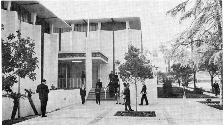
FRONT ENTRANCE —Daylight view of spacious main entrance to new gymnasium. Concrete work and landscaping were all done by Ambassador personnel.
